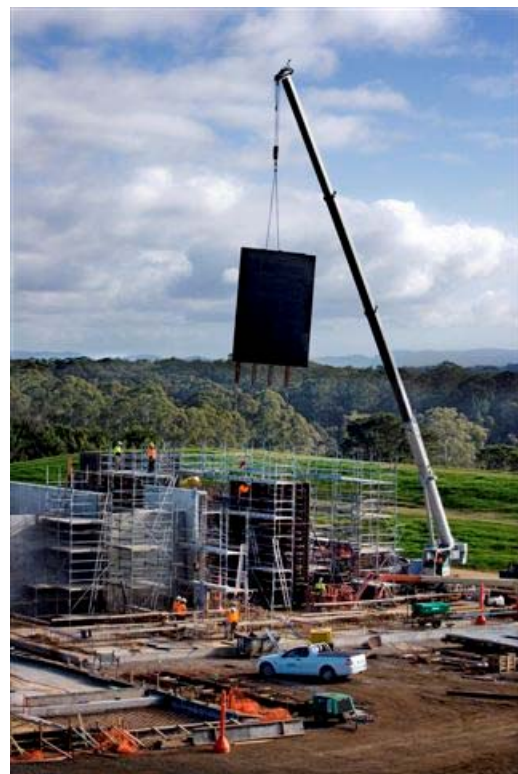
Main treatment building under construction
